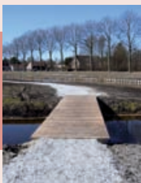
A new bridge improves village access
