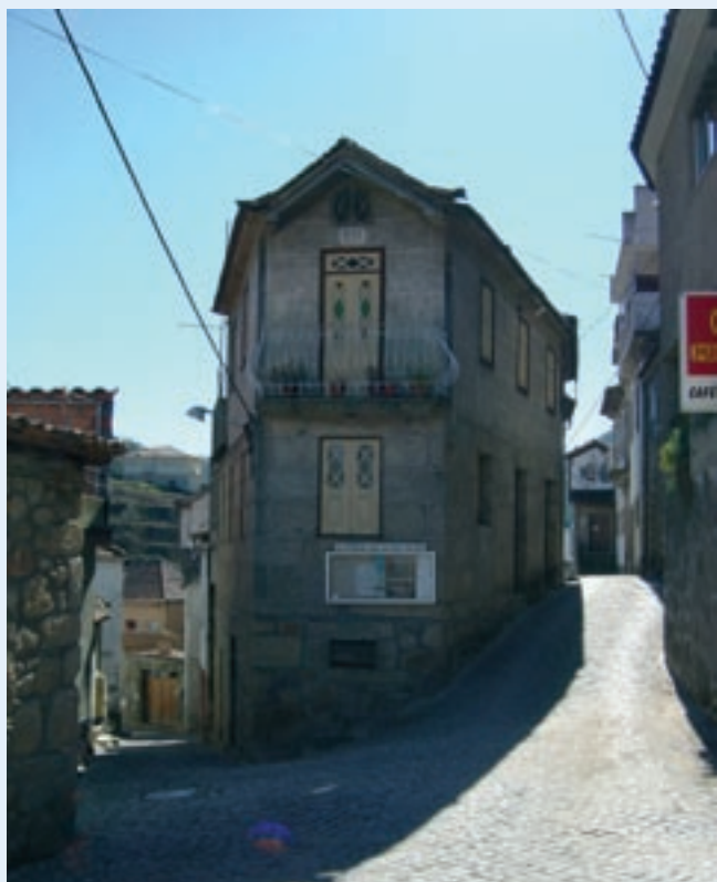
...built with local materials
