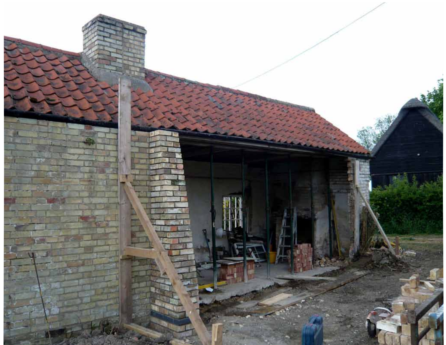
Above Rebuilding the rear wall, with new buttress
